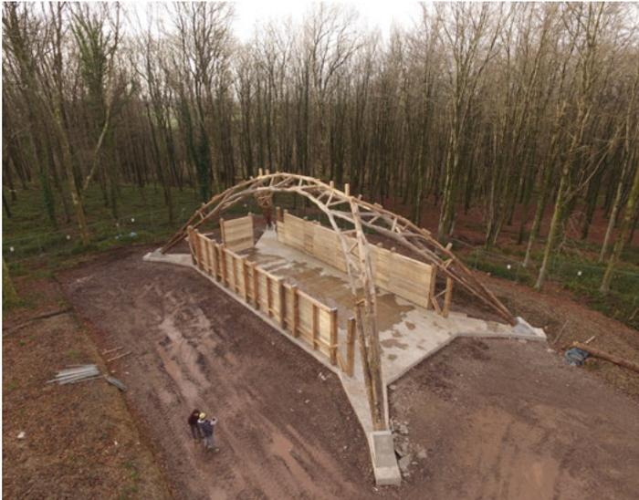
**Figure 1.** The Wood Chip Barn's arching truss.
