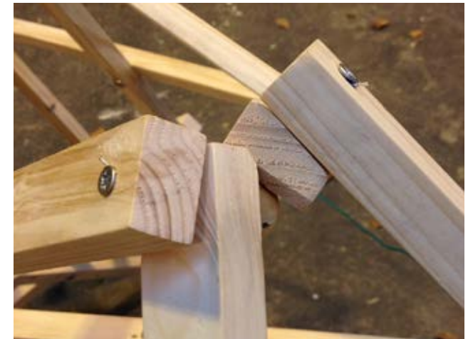
Chamfer closed in arched position
