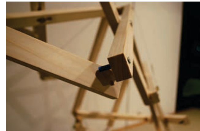
Cable pulled from tubing and screw connection
