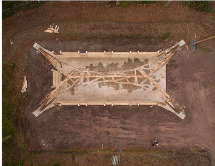
be vertically oriented once the fork was properly positioned above the jig's floor. Corresponding to these points, three square pockets were cut into the 18 sheets of oriented strand board (OSB) by the CNC for each of the 20 forks, a simple vertical support then rising from each pocket to allow the reference points to be precisely set out in X, Y and Z.
