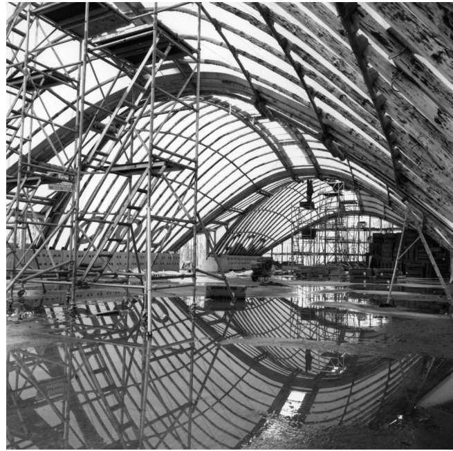
Designed by Richard Burton of ABK and Frei Otto, with the engineers Buro Happold, Hooke Park's main workshop is an impressive long-span enclosure built using low-value material from the surrounding forest. Completed 1989
