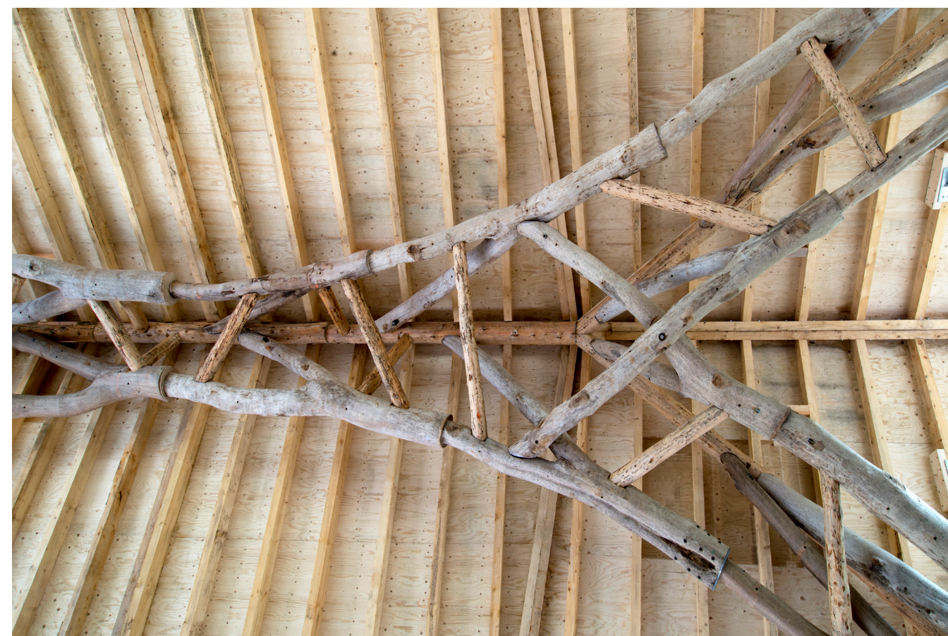
The Wood Chip Barn's robotically fabricated 'tree fork truss' is made of 20 distinct beech forks. Through digital design and fabrication tools the inherent form and structural capacity of the tree is employed directly. Completed 2016
